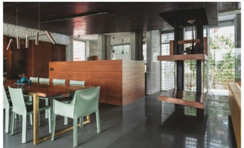
1 The manually powered elevator can transport three people at a time to the upper level by simply paddling like a cycle. This engineering marvel is complete with safety features such as an electrical override.
