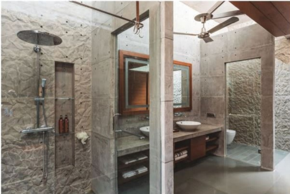
1 Similar to most of the house, the bathroom too is finished in concrete.
