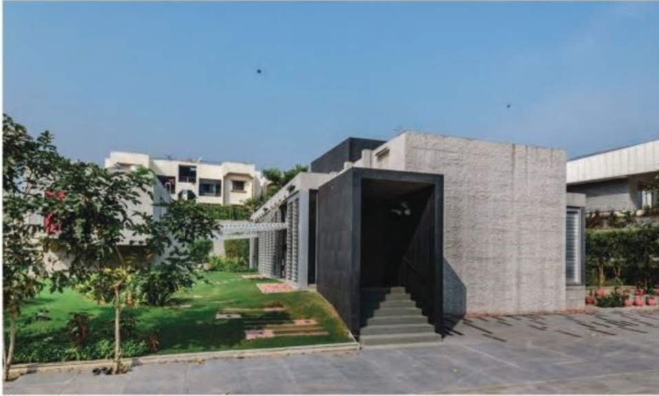
1 Copper tunnel at the textured cube (Living).
