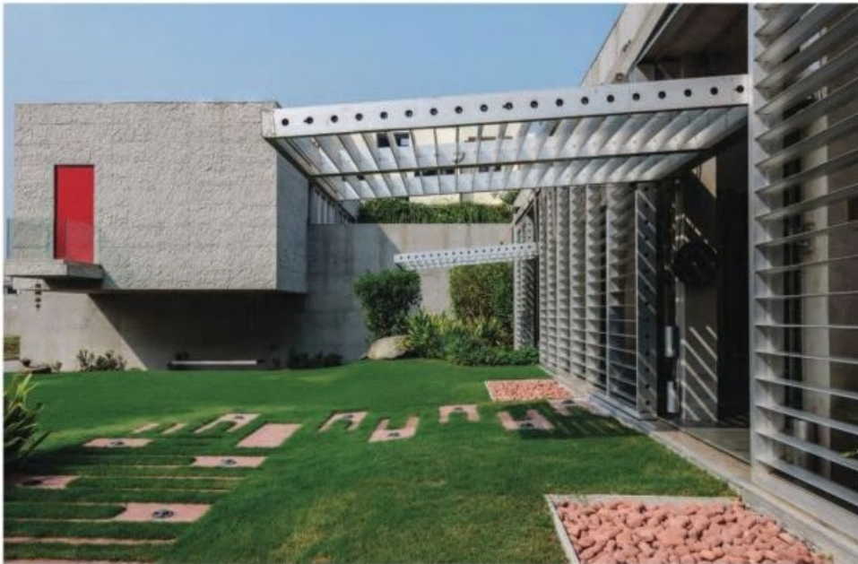
1 All North and South-facing spaces, including the four bedrooms, have indigenously designed operable louvers systems with an open-able layer of glass, from wall to wall.
