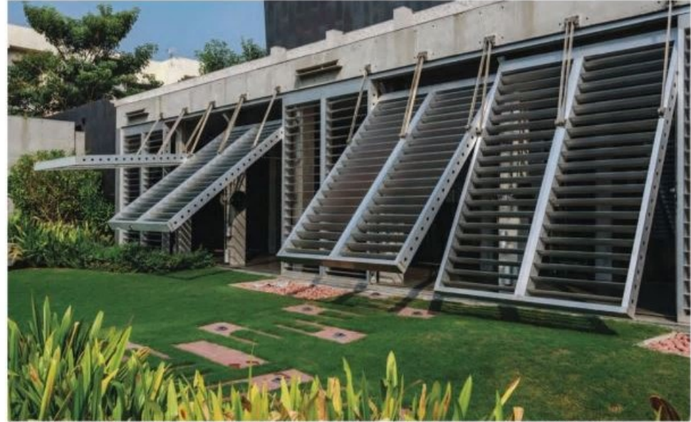
1 The louvers not only come in handy in Surat's hot and humid climate but also help in maintaining the connection with the landscape outside the rooms.
